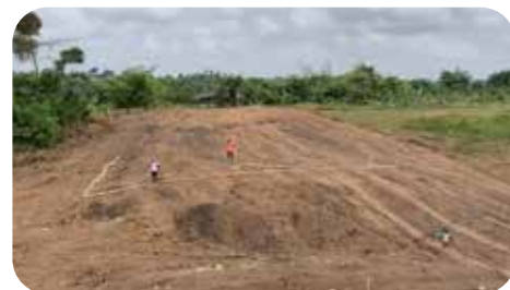
Laying Out the School Perimeter
