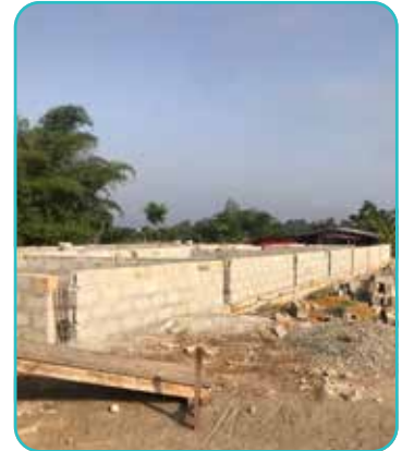
Continuing to Build
